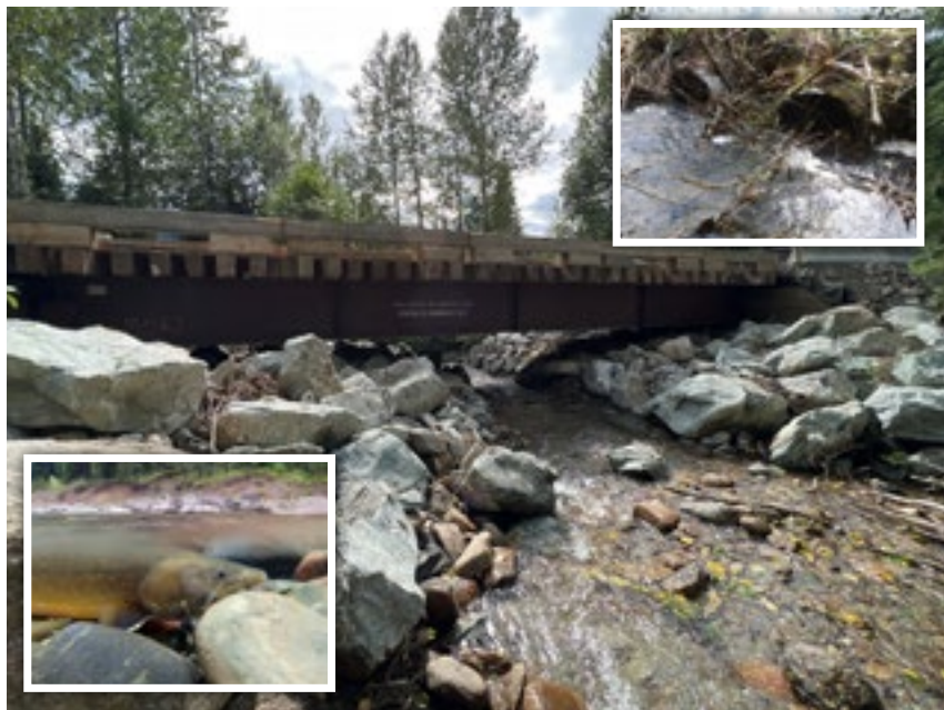
Before (right inset) and after photos of the newly installed bridge. Removal of culverts and installing bridges can improve fish passage for species like bull trout (left inset) in sensitive watersheds. PEA-F23-F-3761-DCA . Photos: New Graph Environment Ltd./ iStock, M. Haring
