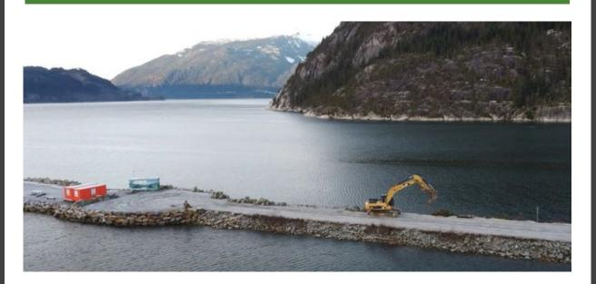
Work to restore fish habitat is underway in the Squamish River Estuary. Since this photo was taken in January, a small section of the spit has been removed, leaving an "island" to the left, and work is progressing to remove more to the right of the excavator. Photo: J. Buchanan
