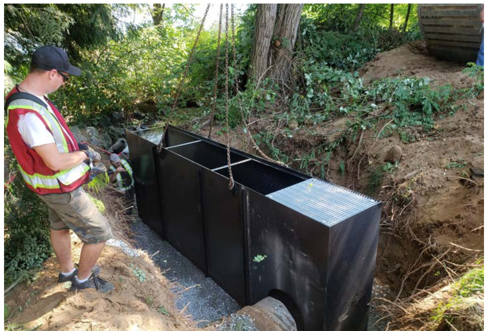
Clockwise from top left: An exclusion fence is set up so that fish can be safely removed from the worksite; the old wooden fish ladder is dismantled; the upper section of the new steel fish ladder is lowered into place. Photos: Fraser Valley Watersheds Coalition
