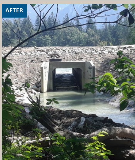
A large concrete box culvert installed in the Squamish River Estuary restored access to juvenile Chinook salmon habitat and resulted in more fresh water in the estuary than there has been for the last 50 years. (COA-F20-F-3067). Photo: Squamish River Watershed Society
