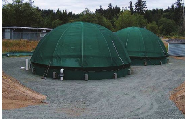
Installation of shade cloth tank covers
