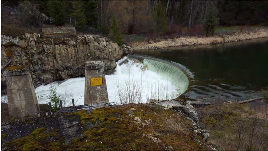
Photo 5. Spillway crest (downstream to the left).
