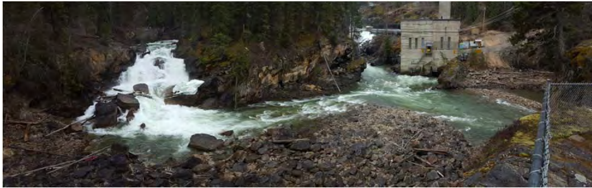
Photo 9. Confluence of spillway flow: spillway channel (left) overflow to old river channel (right).
