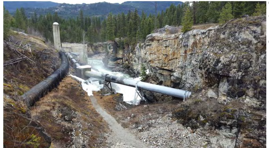
Photo 8. Looking downstream at existing penstocks and old river channel.
