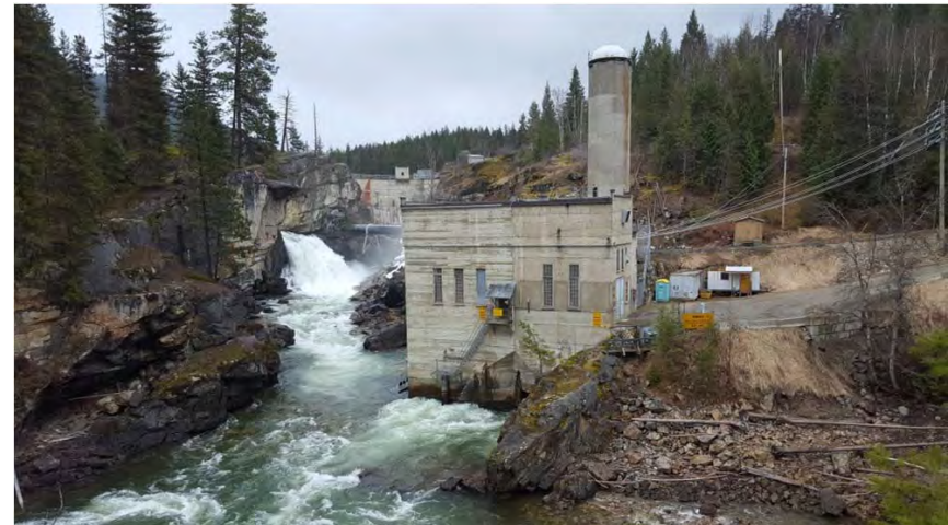
Photo 10. Existing power generation facility with Wilsey Dam in the background. "Bypass pool," to left of structure.
