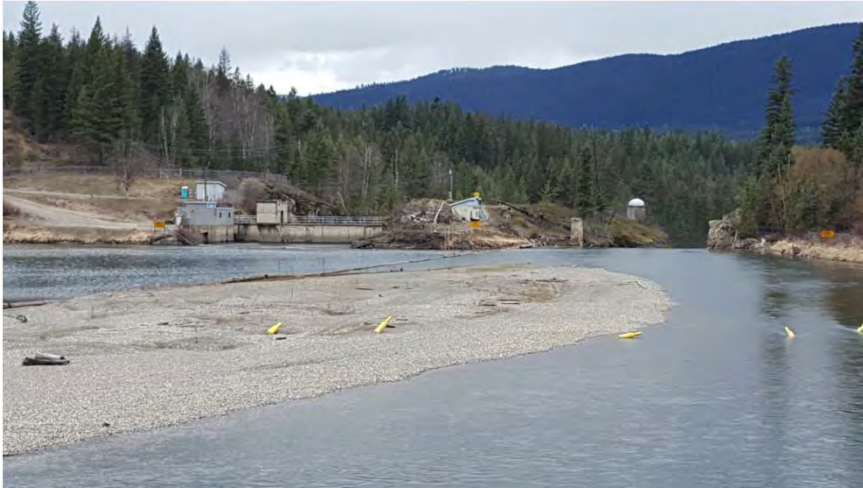
Photo 1. Forebay of Wilsey hydroelectric project looking downstream.
