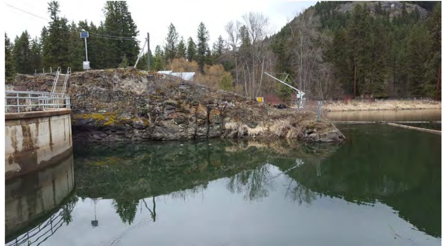
Photo 4. Wilsey Dam (left) and Intake No. 2 (right).
