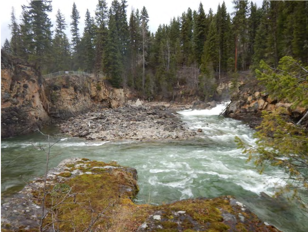
Plate 4: Spillway exit opposite the powerhouse. Powerhouse is located to the right of the photo (source: ONA).
