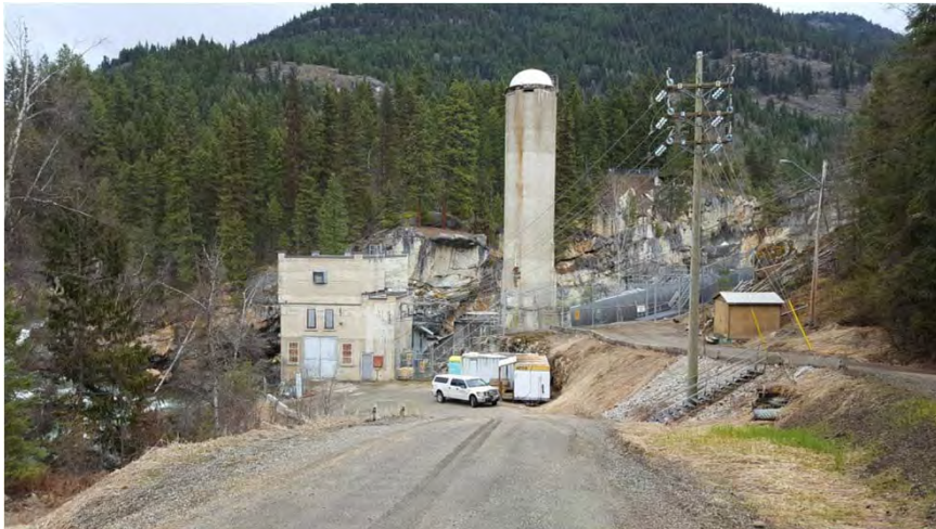
Photo 11. Existing power generation facility and point of downstream access.
