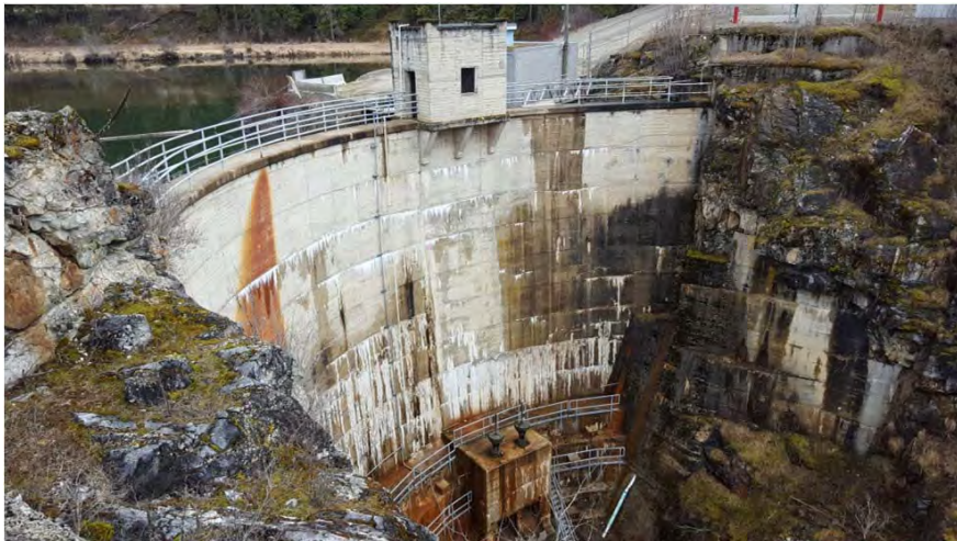
Photo 7. Downstream face of Wilsey Dam concrete arch.
