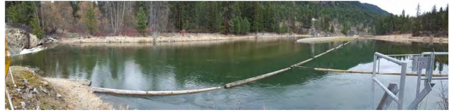
Photo 2. Forebay upstream of spillway crest (downstream to the left). Debris boom in foreground.
