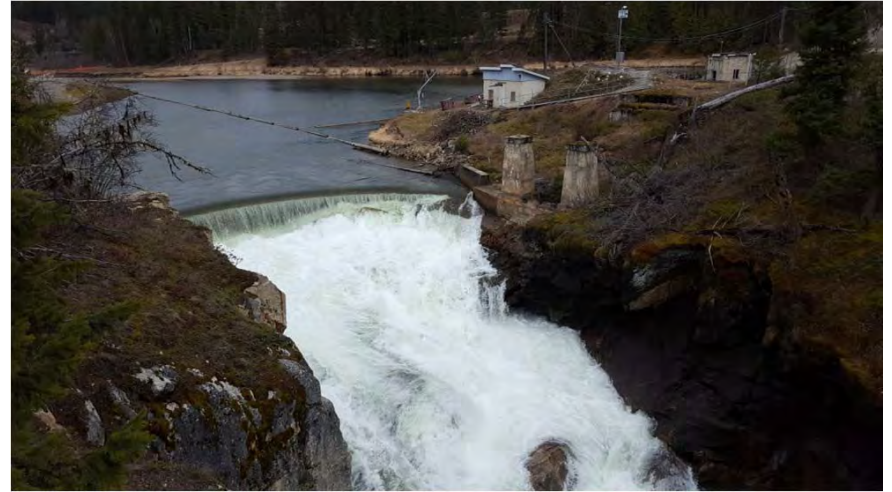
Photo 6. Spillway with forebay in background.
