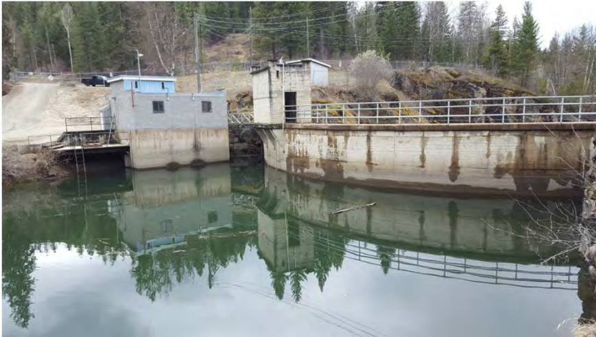
Photo 3. Wilsey Dam structure (right) and Intake No. 1 (left).
