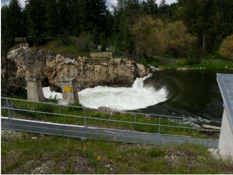
Plate 2: Wilsey Dam spill crest (source: BC Hydro).
