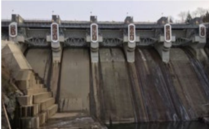
Ruskin Dam, in the Stave River Watershed, is one of 31 dams the FWCP is working to compensate for. Six new panels were installed on the dam in 2019, thanks to Kwantlen First Nation’s artist Brandon Gabriel. Photo: BC Hydro.
