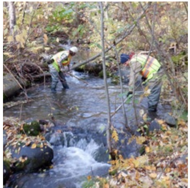
Murphy Creek Spawning Channel is 225 metres long and features 28 gravel-filled step pools that are cleaned each fall in preparation for the next spawning season. COL-F23-F-3764 . Photo: A. Mallette.
