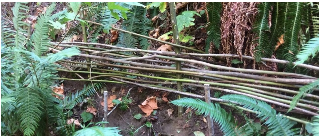
Sites identified to have steep eroding banks were treated with wattle fences. Photo: A-Tlegay Fisheries Society and Ecofish Research Ltd.
