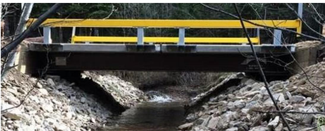
UKEEP funded several fish passage improvement projects, including removing a culvert and [installing a bridge span at Wickman Creek](#). Photo: Evan Kleindienst, VAST Resource Solutions.
