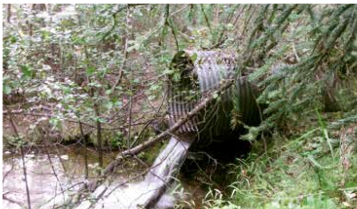
Perched culvert acting as a barrier to fish passage in the Finlay Arm watershed. (photo: Ecofor Consulting)
